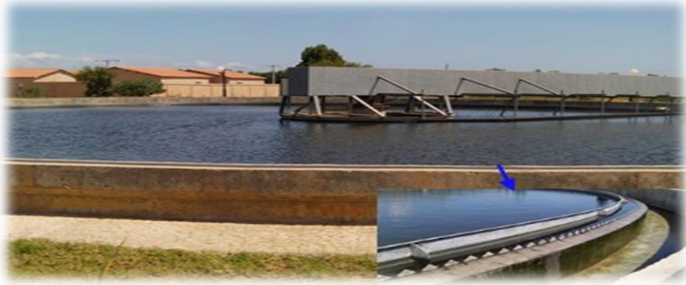
Figure III.10 : Clarificateur.
