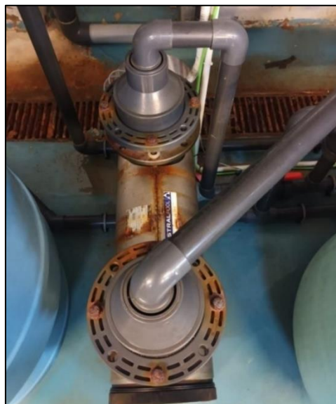
Figure8 . UV sterilizer in the pre-fattening room (CNRDPA)
