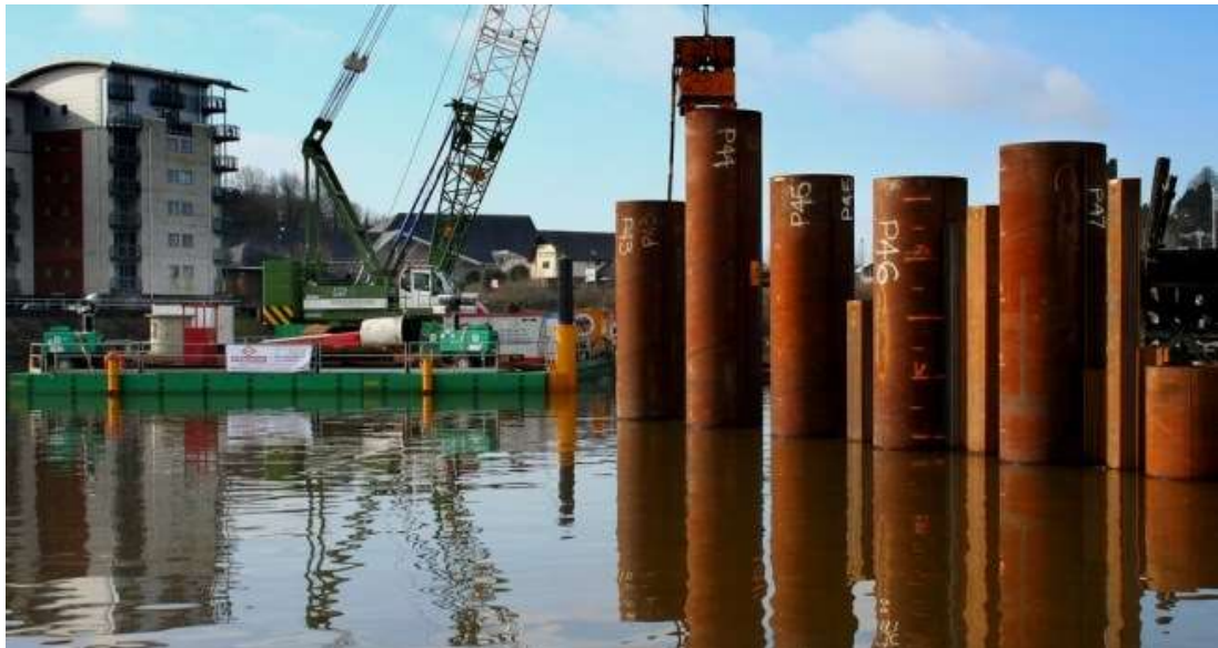
Figure 8: Pieux métalliques (nicolas, n.d.)
