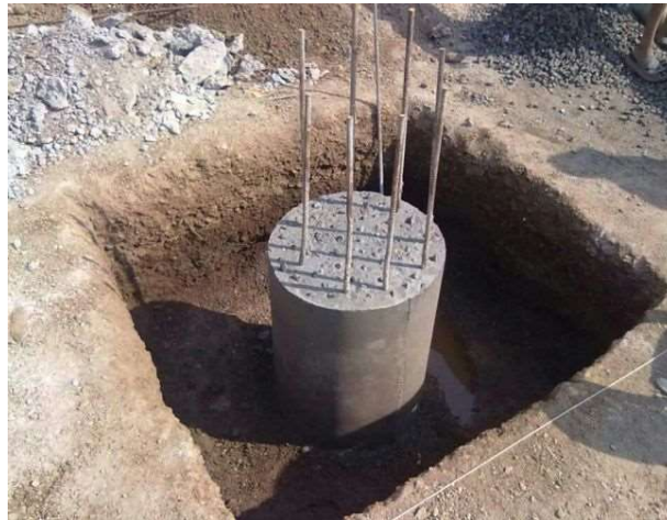
Figure 7 : Pieux en béton coulés en place [ https://bouassidageotechnics.com/2017/02/27/conventional-methods-estimating-the-settlement-of-single-piles/ ]
