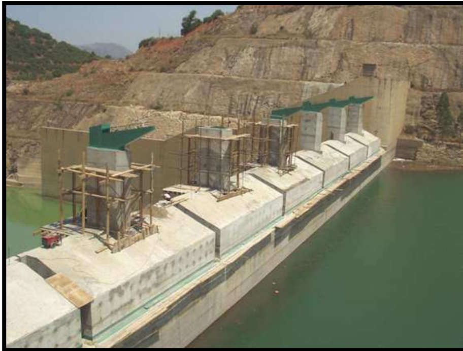
Figure .II.13. Barrage Beni Amrane
