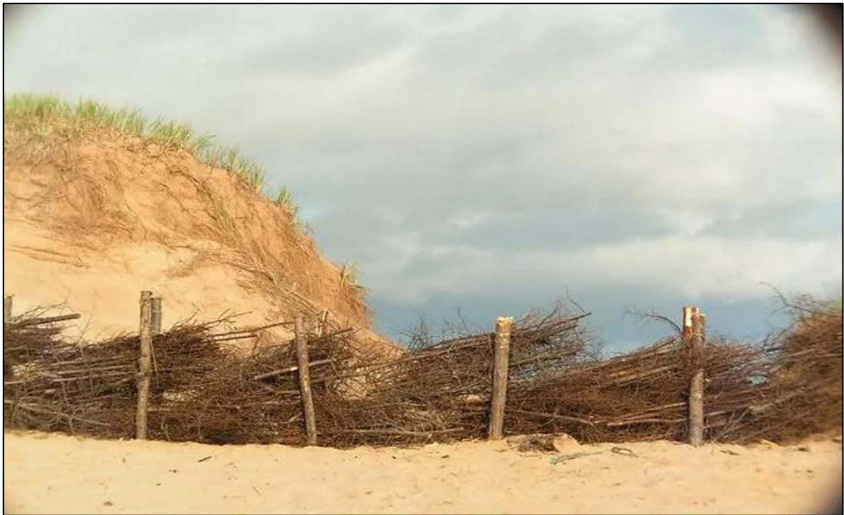
Figure 40: photo de fascine (Attention fragile, 2021)
