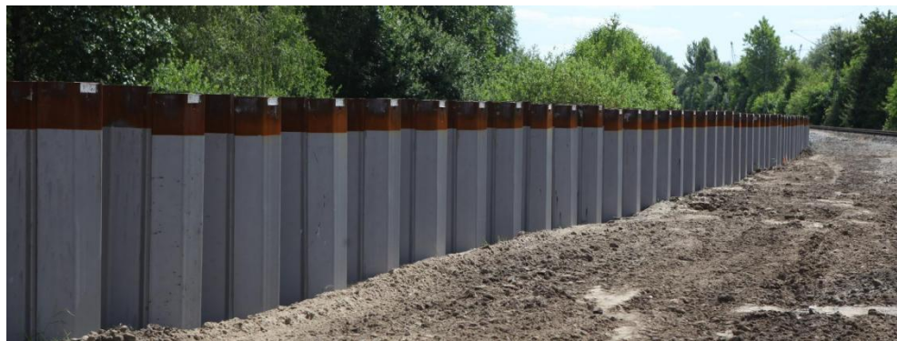
Figure 7: Steel sheet pile sections.(U Sections | ArcelorMittal Sheet Piling, n.d.)
