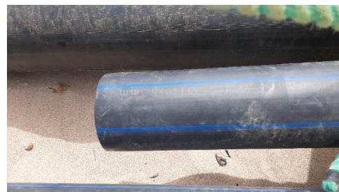
Figure 26: Tube HDPE de 315 mm.
