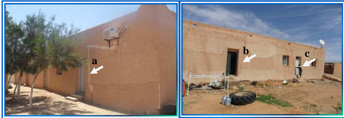
Figure II.27 : Base de vie
