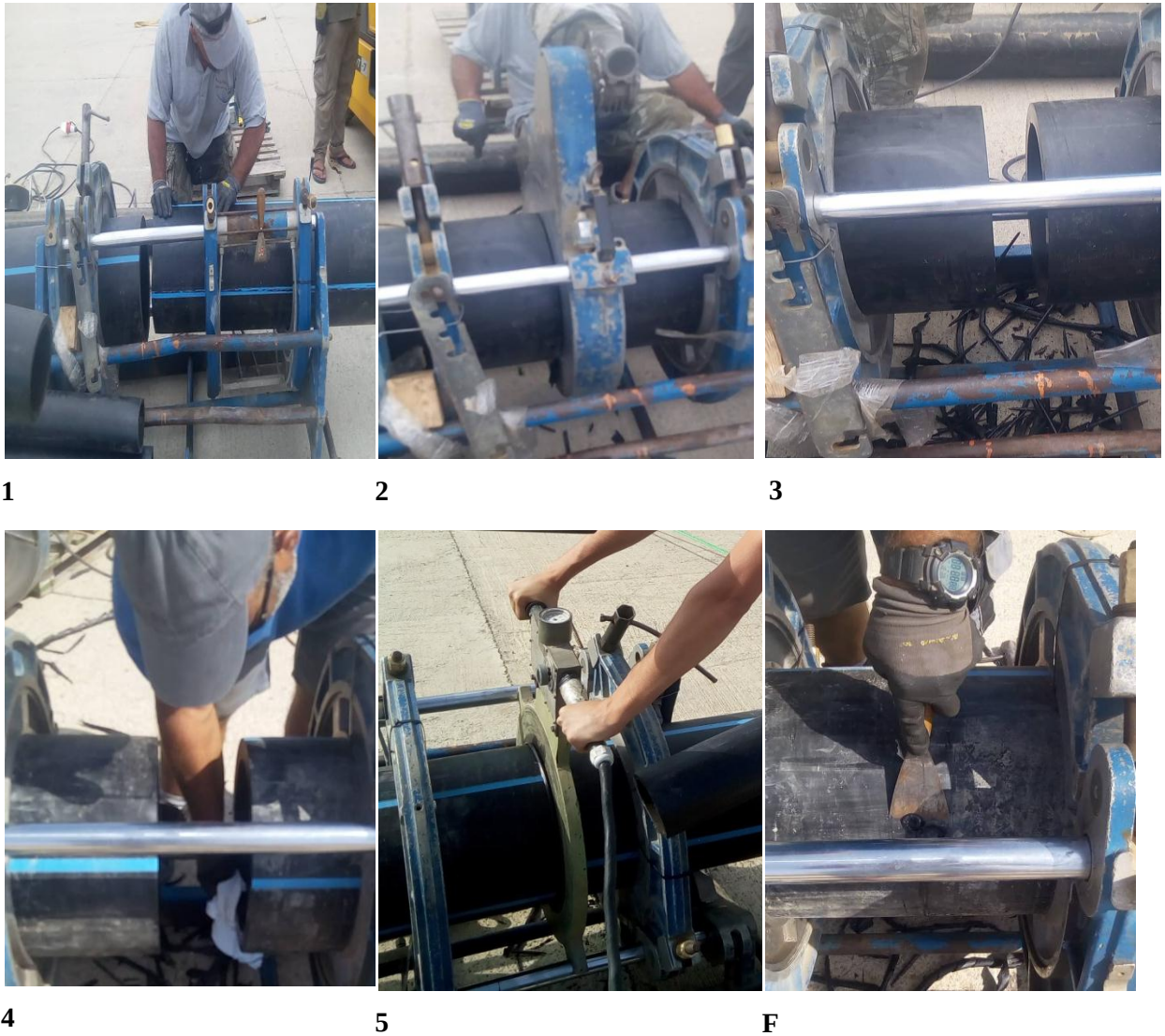
Figure II. 13. Le soudage des tuyaux (Sahraoui,2019)
