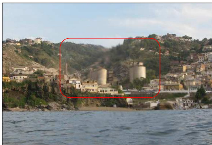
Figure II.4: Cimenterie de Rais Hamidou (Photo : LAMOUTI, 2011)
