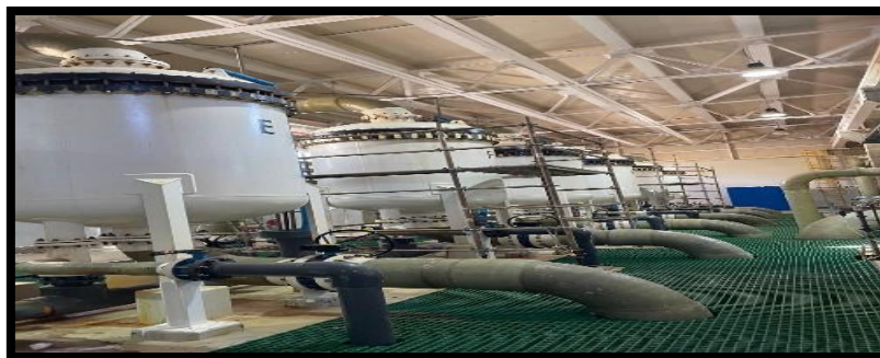
Figure III.16: Filtres à cartouches.
