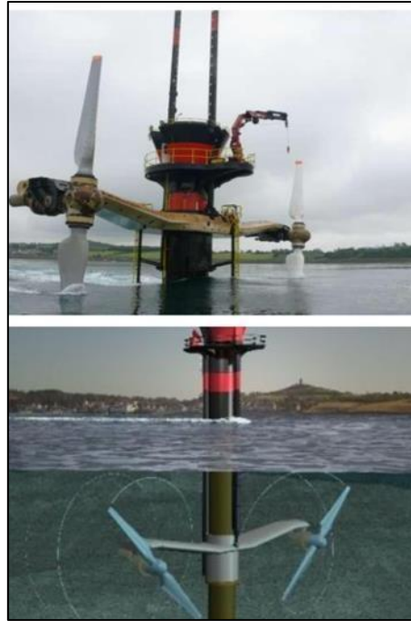
Figure 4: The Seagen 1.2 MW device operating at Strangford Lough, Northern Ireland (U.K.)
