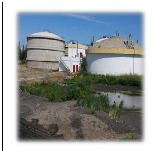
Figure III.10 : Digesteurs
