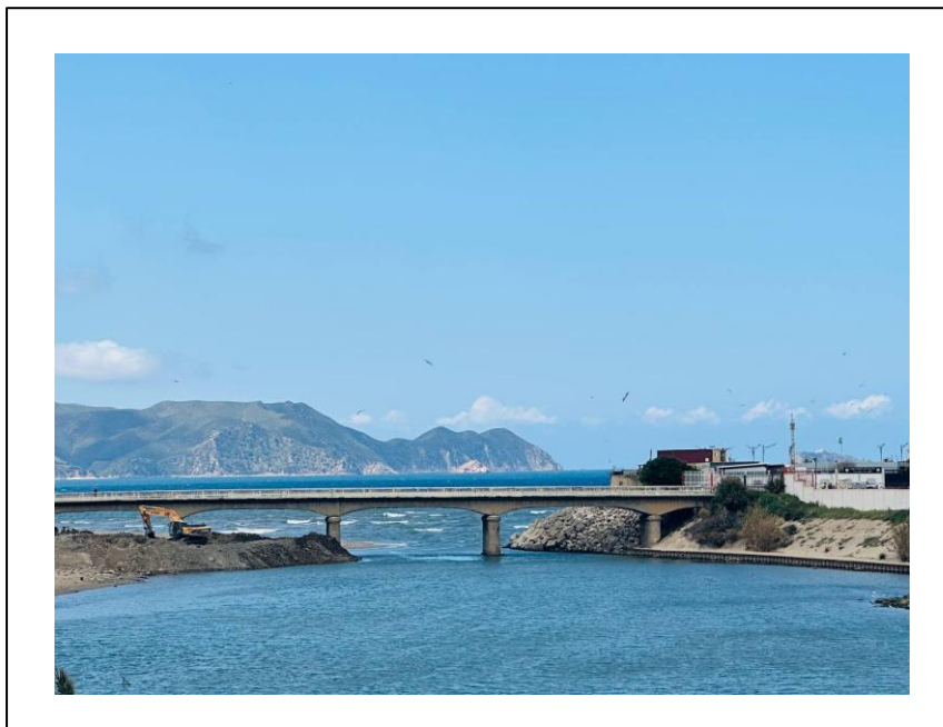
Figure 95: Image of the bridge studied over Oued Saf-Saf.
