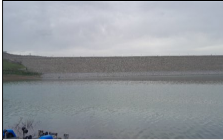
Figure 5. El Maouane Dam, Sétif Province, Algeria.
