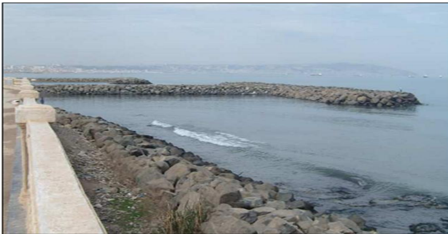
Figure II. 2: Protection de front de mer.
