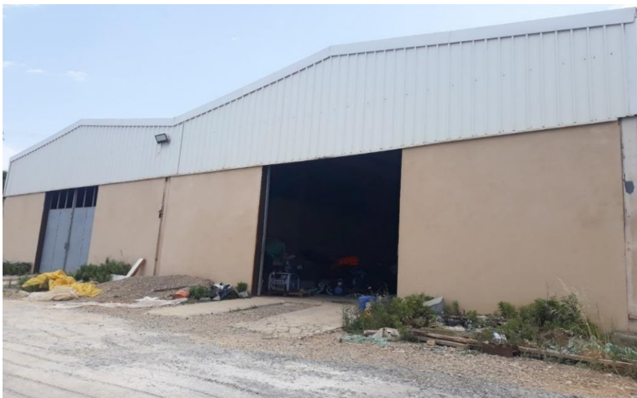
Figure II. 3: Hangar de stockage (Sarl Aqua Cap, 2021).
