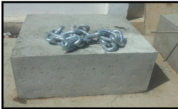
Figure 35: Un corps-mort.
