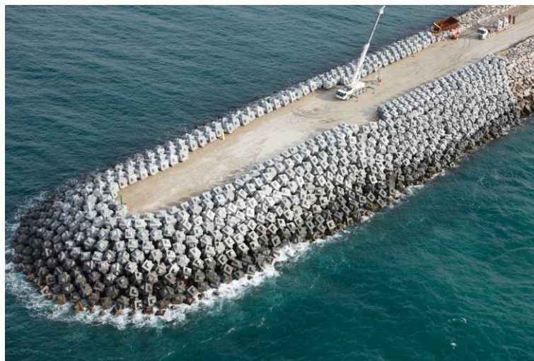
Figure 6: Rubble-mound breakwater during armor layer construction
