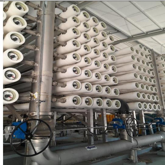
Figure 12: Tubes de pression d'osmose inverse
