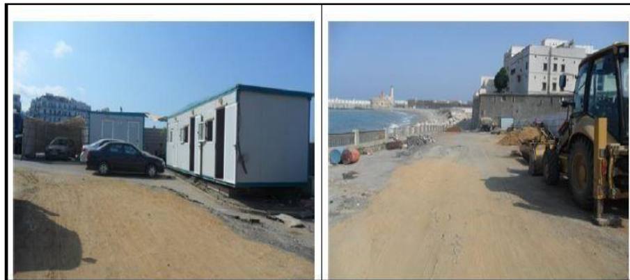
Figure 72: Installation du chantier
