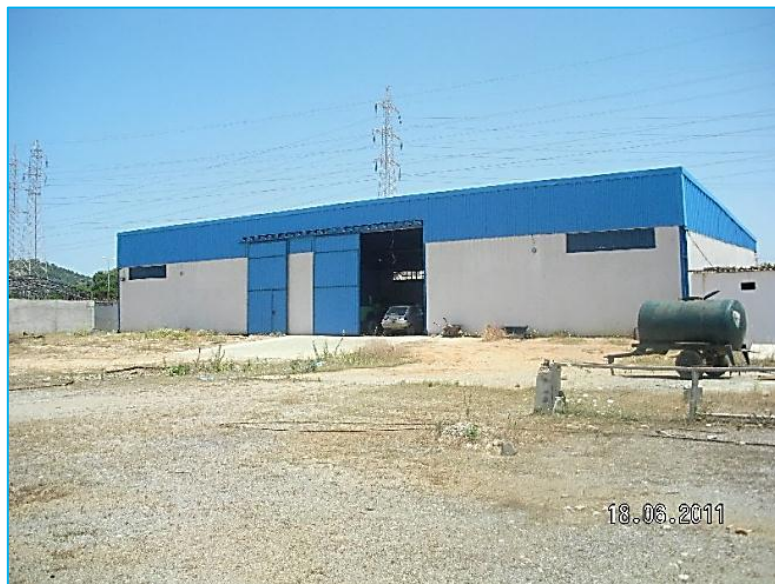
Figure 48 Magasin de stockage
