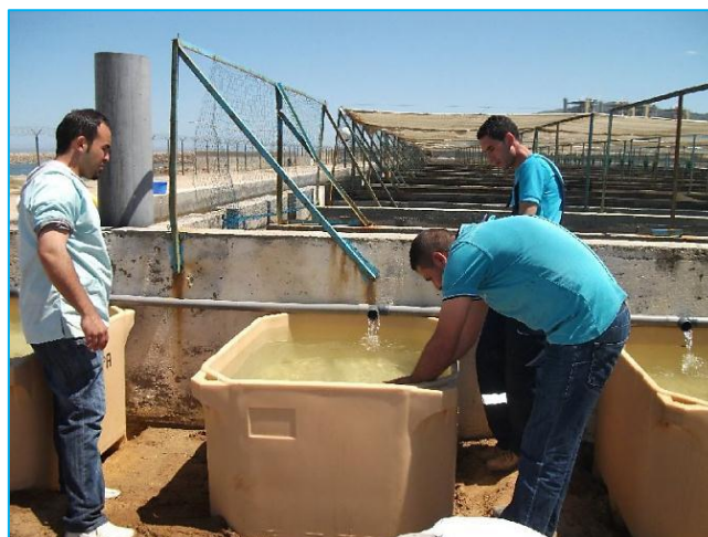
Figure 71 Installation des bacs
